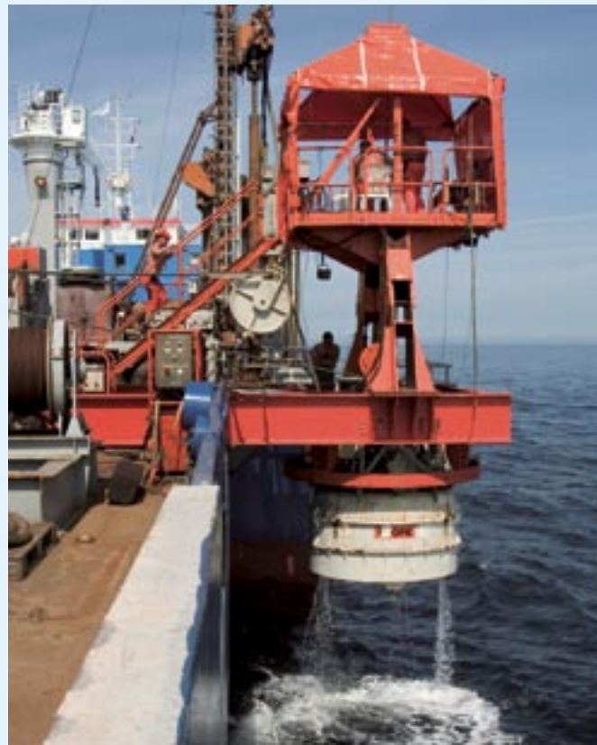
GEO's CPT rig, SCOPE.
